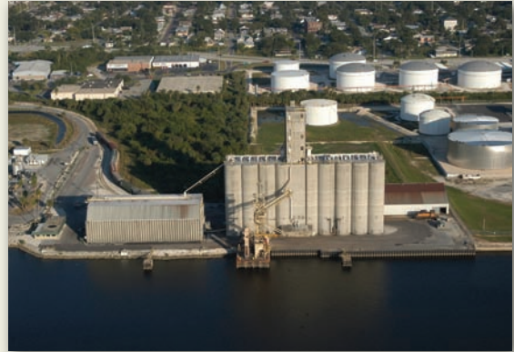
Cargill's Tampa port grain elevator
