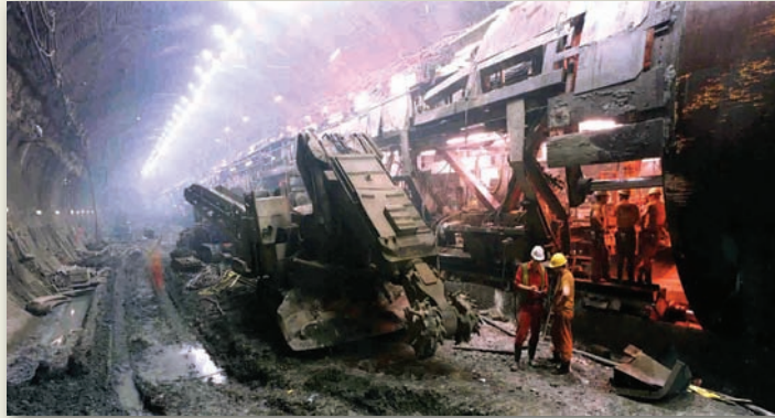
Construction of the Chunnel
