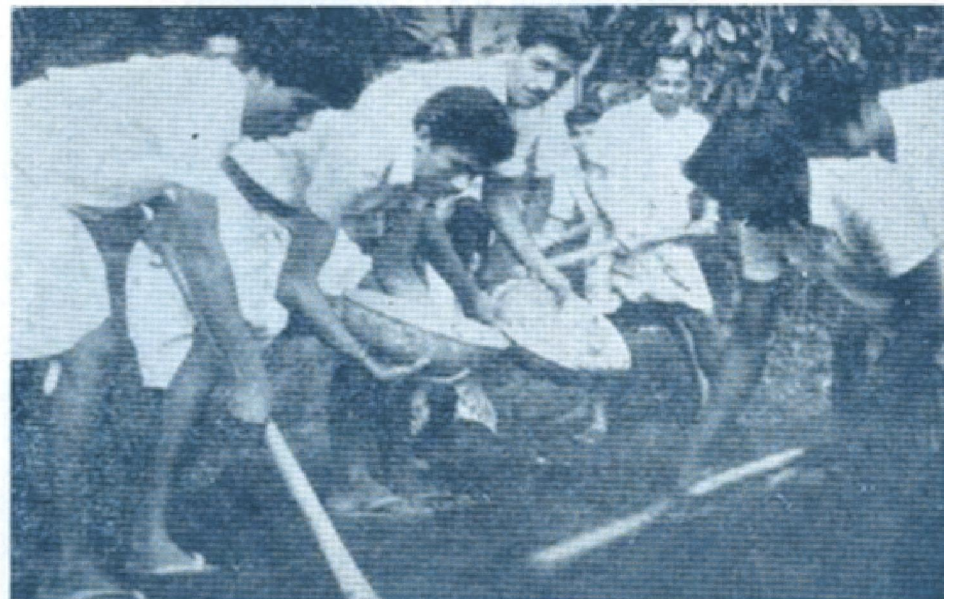
Planning Forum Members on Road Construction Work
